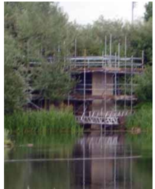
Berkeley Bat House, while under construction, seen across the Sheltered Lagoon
